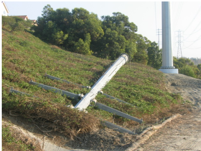
Figure 2 – Dismantled steel poles are cut up and removed from the right-of-way.
