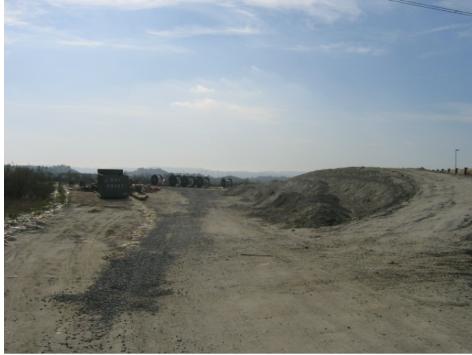
Figure 1 – The spoils pile behind the Viejo Substation will be removed or stabilized.
