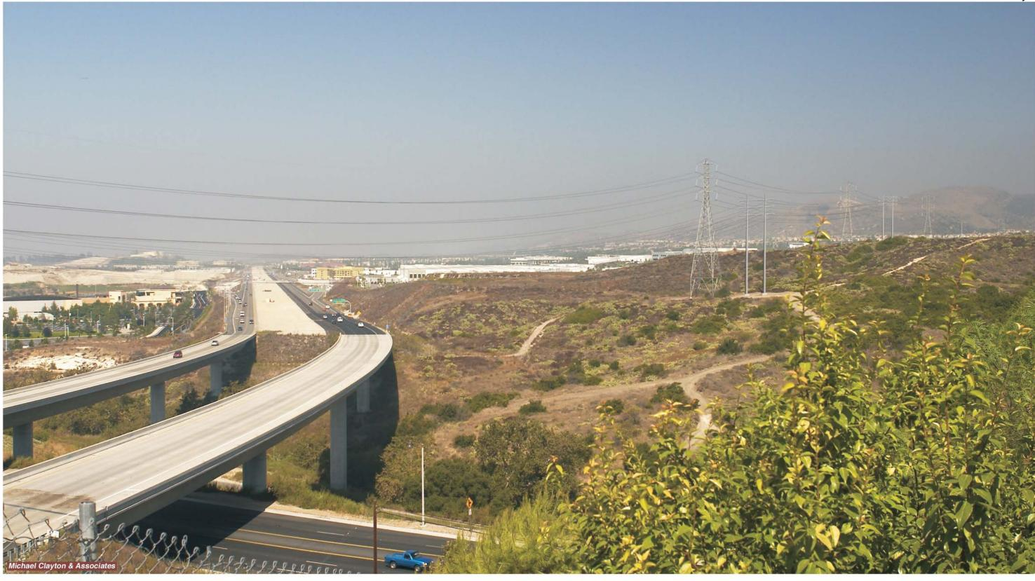
A visual simulation of the proposed project from Key View Point 4 within a residential development along Painted Trails. This view is to the northwest toward proposed tower locations HF-11 (closest) and HF-12. As shown in the simulation, the proposed H-Frame structure with their double poles and multiple, horizontal cross-members are noticeably more prominent than the existing single pole 66 kV towers that are to be replaced.
