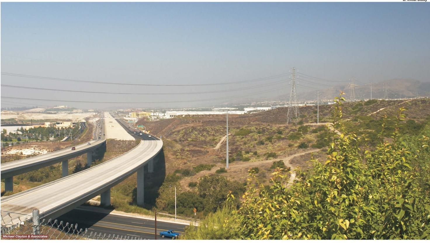
The **existing view** to the northwest from Key Viewpoint 4 within a residential development along Painted Trails. This view encompasses the existing M2-P4 (closest), M2-P5, and M2-P6 66 kV tower locations and the span to the south over SR 241. The M2-P4 structure would be eliminated and the M2-P5 and M2-P6 single-pole structures would be replaced with the corresponding double-pole H-Frame 66 kV towers HF-11 and HF-12
