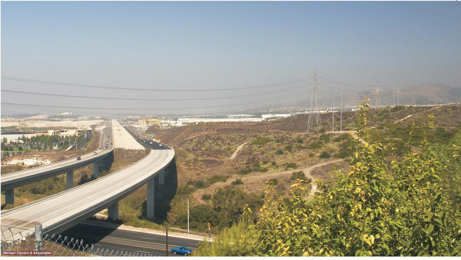
A visual simulation of the proposed project from Key View Point 4 within a residential development along Painted Trails. This view is to the northwest toward proposed tower locations HF-11 (closest) and HF-12. As shown in the simulation, the proposed H-Frame structure with their double poles and multiple, horizontal cross-members are noticeably more prominent than the existing single pole 66 kV towers that are to be replaced.
