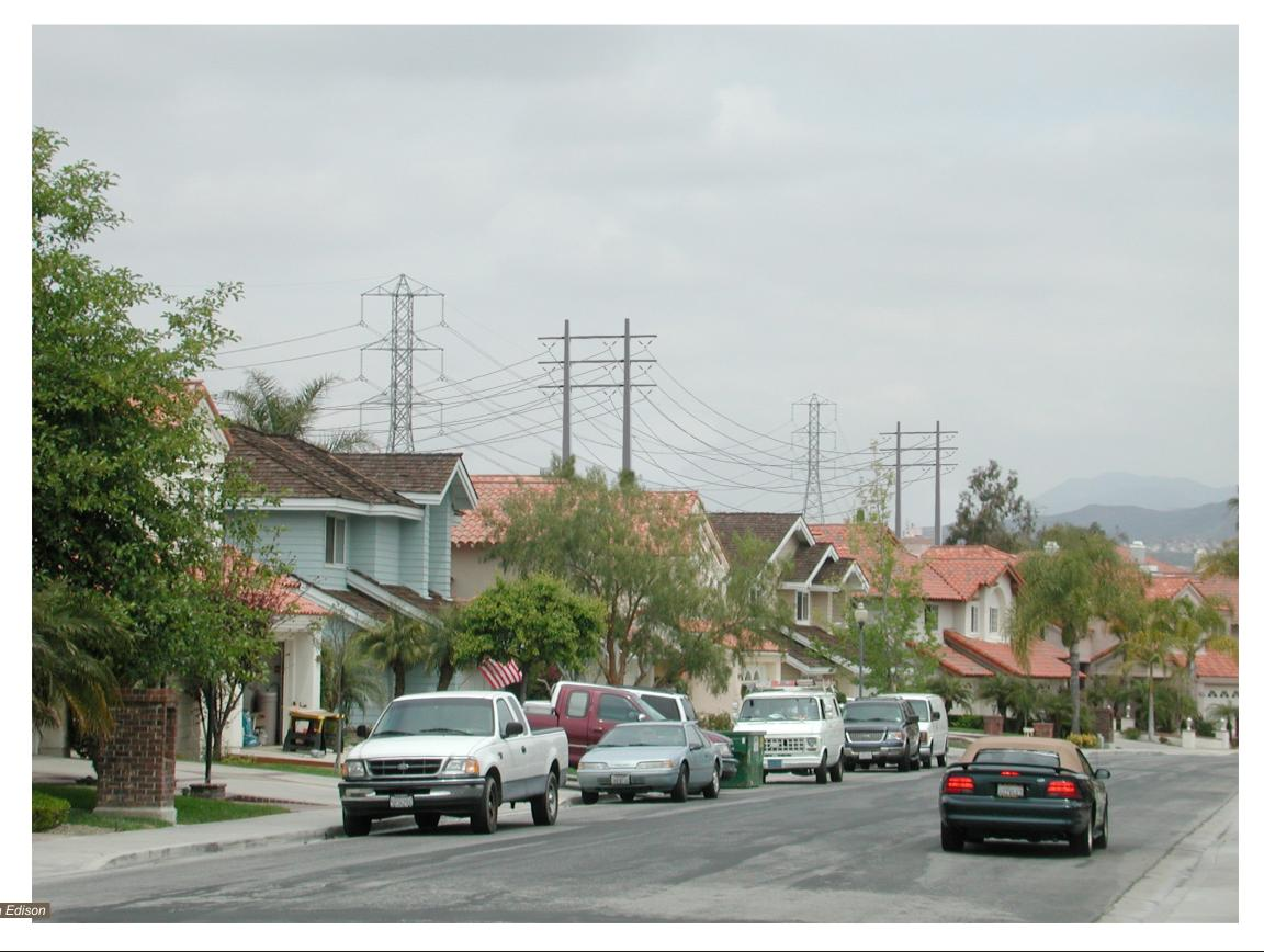
A visual simulation of the proposed project from Key Viewpoint 8 from a residential driveway on the east side of Wayside. This view encompasses the proposed 66 kV H-Frames HF-06 and -07, as well as the existing 220 kV towers M21-T2 and -T3. As shown in the simulation, the proposed structures would appear larger than the existing 66 kV poles, but still smaller than the existing 220 kV towers.
