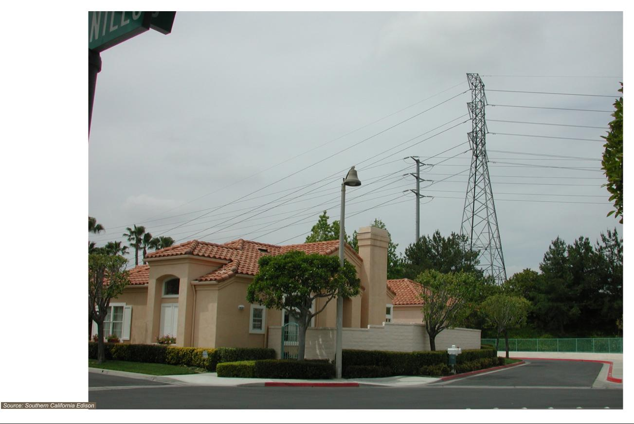
The existing view to the west from Key Viewpoint 7 from neighborhoods east of the proposed project. This view encompasses the existing 66 kV pole M1-P5 as well as the existing 220 kV tower M22-21. This 66 kV single-pole structure would be replaced with H-Frame HF-08.
