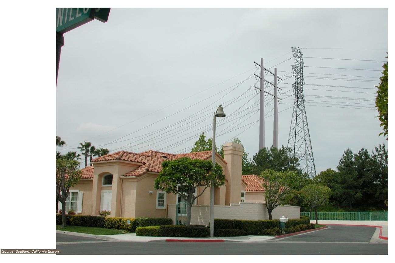
A visual simulation of the proposed project from Key Viewpoint 9 from neighborhoods east of the proposed project. This view encompasses the proposed 66 kV H-Frame HF-08 as well as the existing 220 kV tower M22-21. As shown in the simulation, the proposed H-Frame would be larger than the existing 66 kV pole, but distinctly smaller than the existing 220 kV tower. Just out of view, three existing 66 kV poles (M1-P3, -P4, and P6) would be removed and not replaced.
