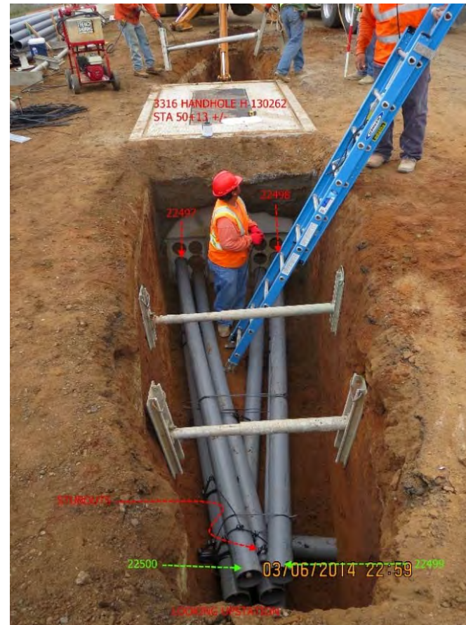
B. Typical 12-kV Duct Bank
