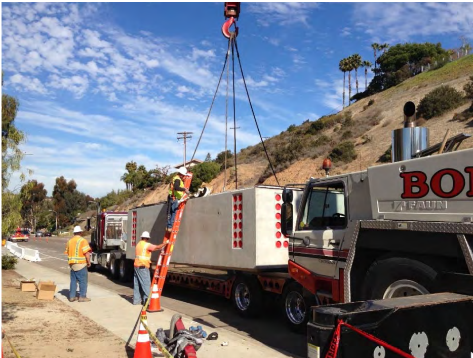
C. Typical Type 3327 Vault
