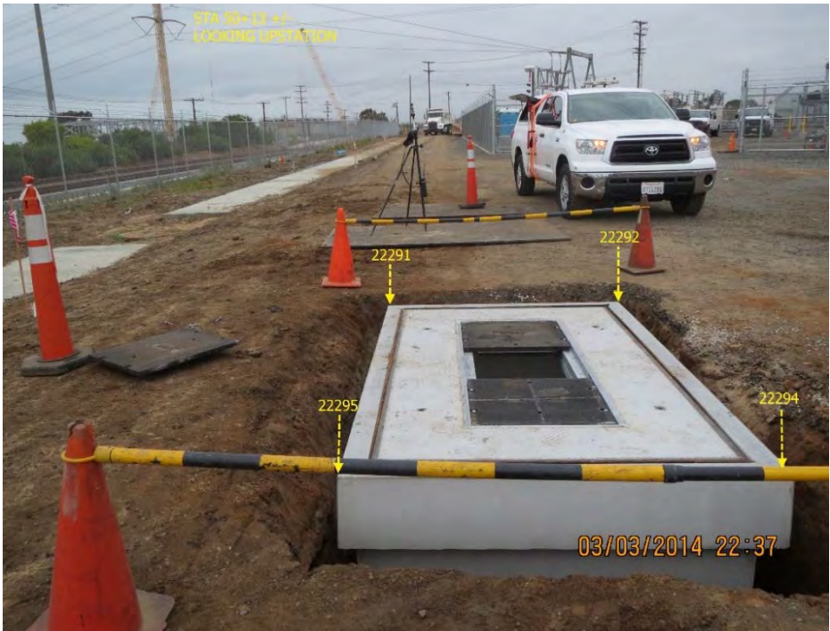
D. Typical Vault Installation
