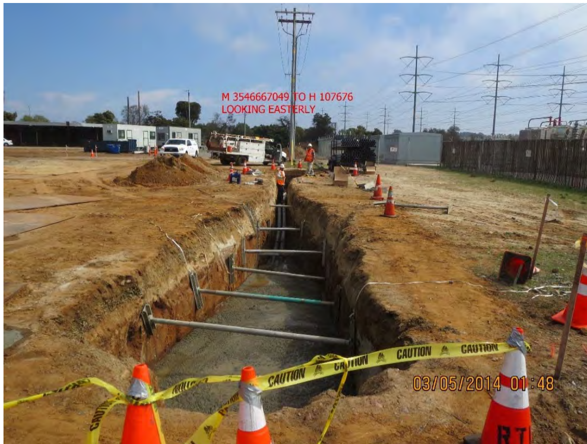
A. Typical 12-kV Trench
