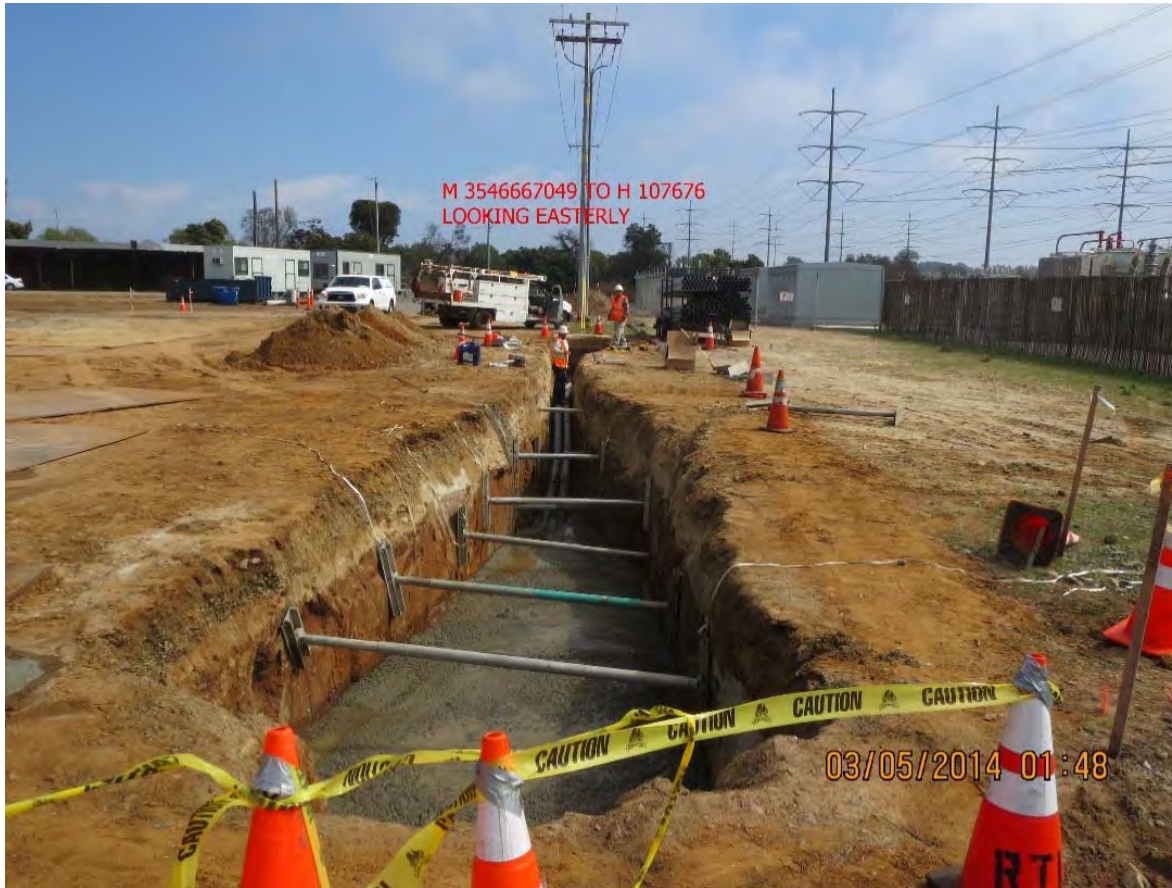
A. Typical 12-kV Trench
