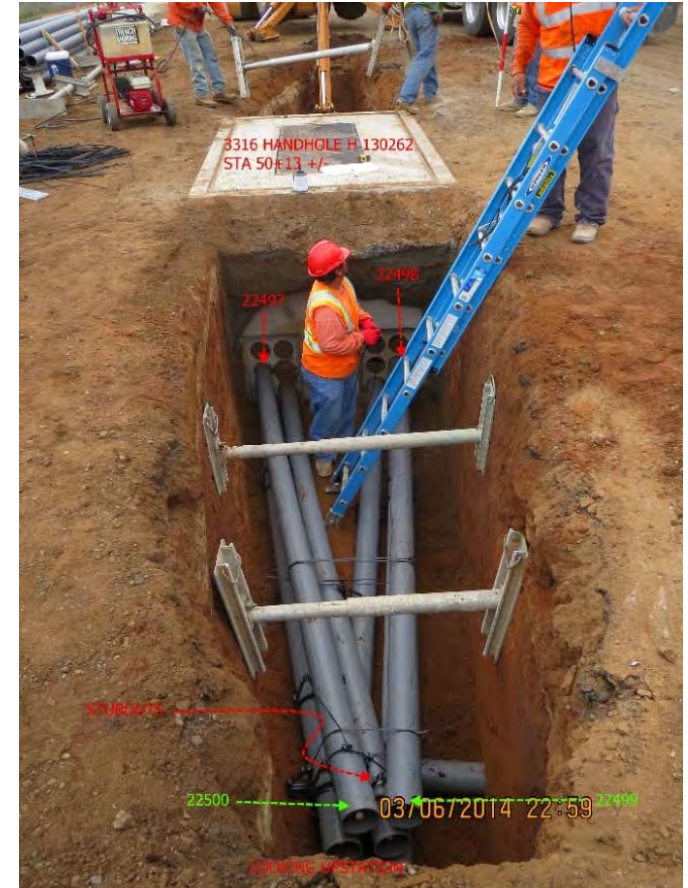
B. Typical 12-kV Duct Bank
