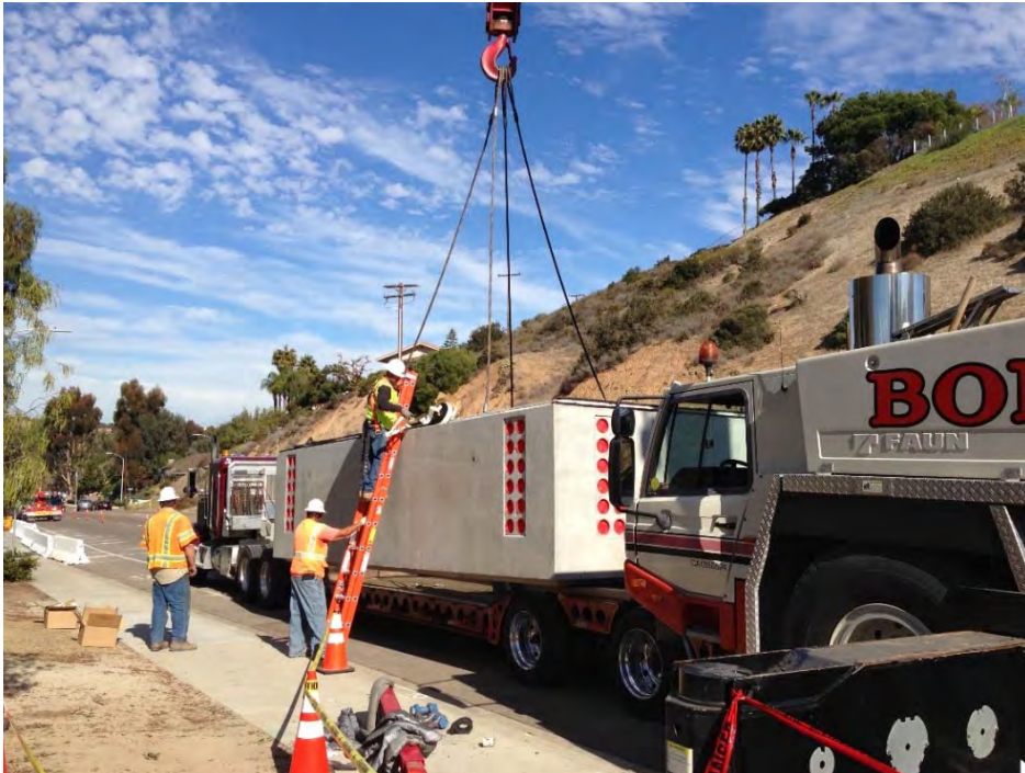
C. Typical Type 3327 Vault
