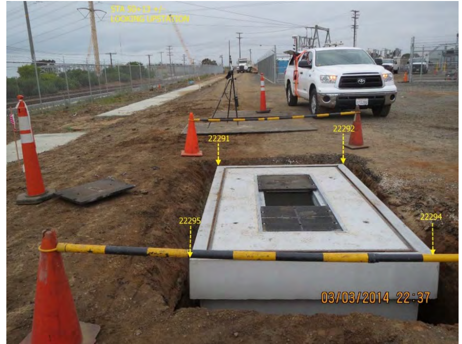
D. Typical Vault Installation
