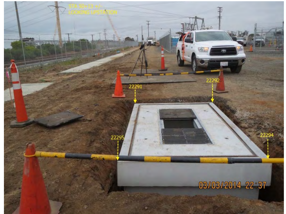
D. Typical Vault Installation
