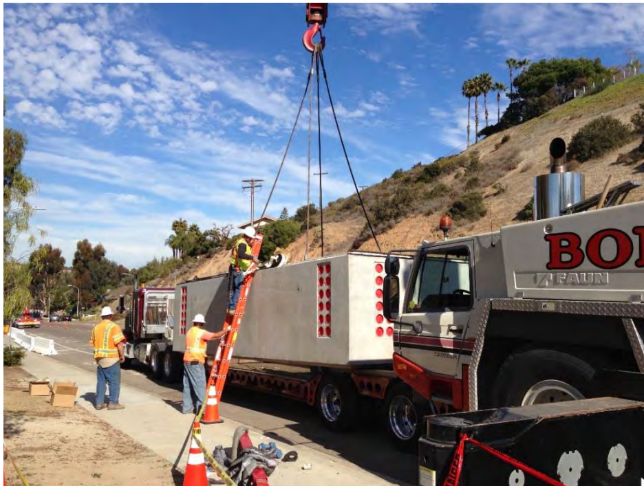
C. Typical Type 3327 Vault
