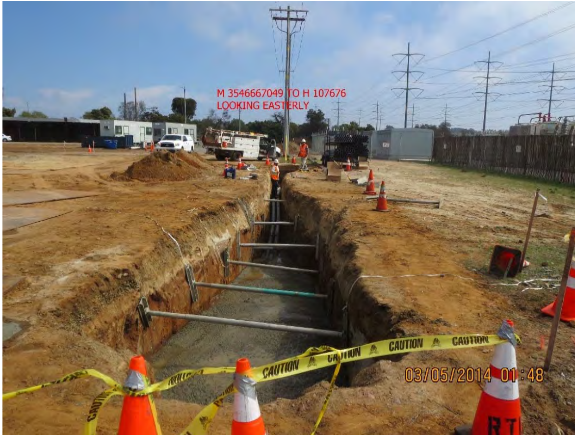
A. Typical 12-kV Trench
