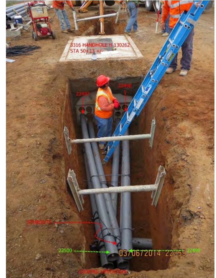
B. Typical 12-kV Duct Bank
