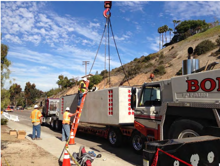
C. Typical Type 3327 Vault
