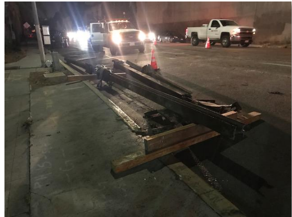
Photo 15. Salvage of historic trolley tracks encountered during excavation on Kettner
