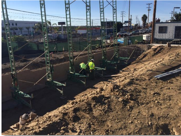
Photo 5. Construction of the perimeter substation wall
