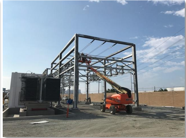
Photo 6. Construction of the interior substation components
