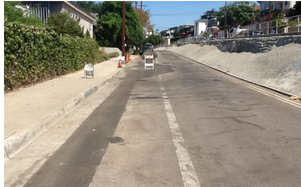
Photo 11. Paving of the trenchline after construction along Columbia Street
