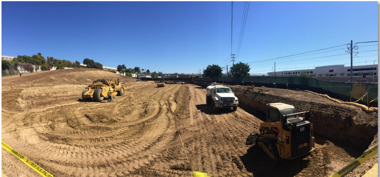
Photo 4. Grading of the substation site
