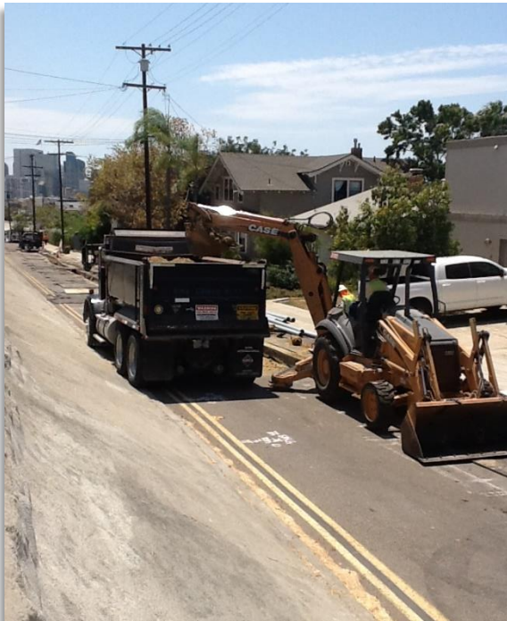
Photo 8. Trenching operations along Columbia Street occurred during daylight hours
