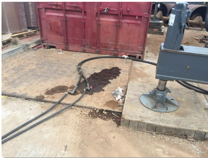
Photo 18 (above). Leaking hydraulic hoses at the jack and bore location
