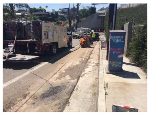
Figure 1 – Crews saw-cutting along Columbia Street in advance of trenching crews.
