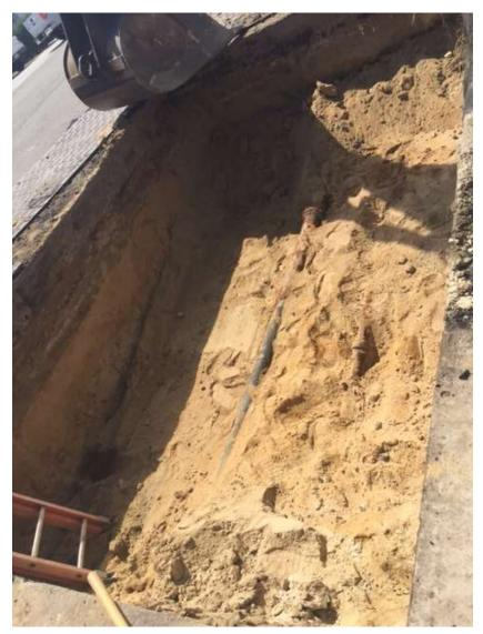
Figure 3 – Abandoned utility pipes found during vault excavations along Columbia Street.
