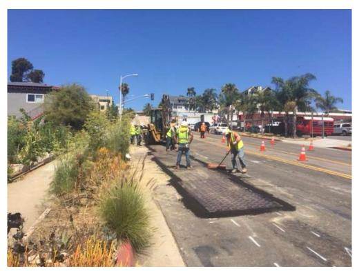
Figure 2 – Steel plate placement over the trenchline at the end of the day along Laurel Street.
