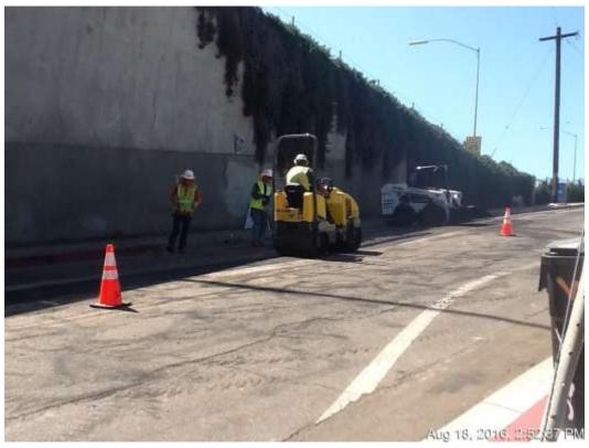
Figure 4 – Temporary paving of the completed trench, Columbia Street 12-kV Underground.
