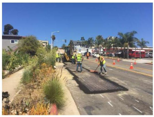
Figure 3 – Trench backfilling and clean-up activities along W. Laurel Street, 12-kV Underground.
