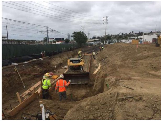
Figure 2 – Form construction and rebar installation for the perimeter wall footing.
