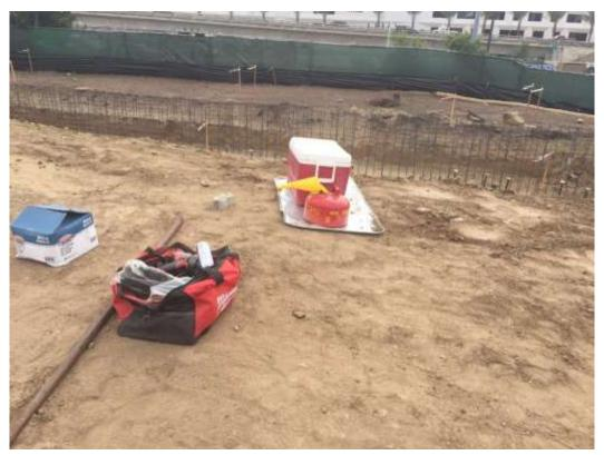
Figure 4 – Crews placed the generator and gas can on top of a drip pan to avoid any contamination to the ground.
