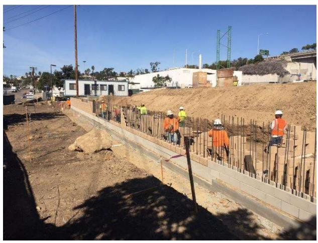
Figure 2 – Block wall installation along the southwestern site boundary.
