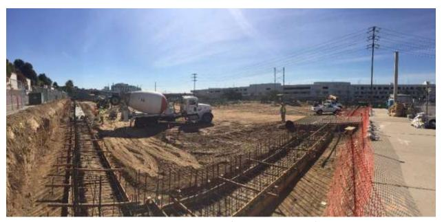
Figure 1 – Concrete placement of the perimeter wall footing.
