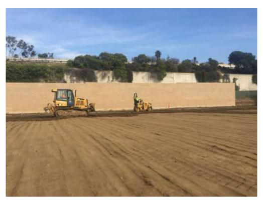
Figure 1 – Construction contractor preparing the ground surface prior to the rain event in order to minimize accumulation of storm water on the site.
