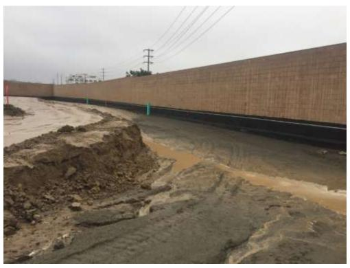
Figure 2 – Storm water drained into the lower corner of the site and into the drain system.
