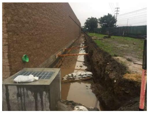
Figure 3 – Location of the storm water accumulation adjacent to the block wall footing (during the storm event).
