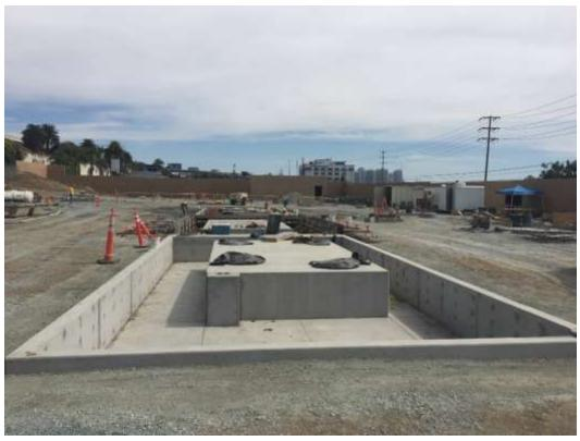
Figure 1 – DCX crews constructed the oil containment area surrounding the transformer pads.
