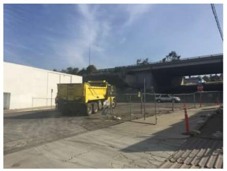
Figure 4 – Hauling of excess soil for disposal; haul trucks covered the loads prior to leaving the substation site.
