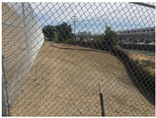
Figure 5 – Temporarily disturbed area adjacent to the railroad right-of-way; SDG&E is assessing possible stabilization treatments.
