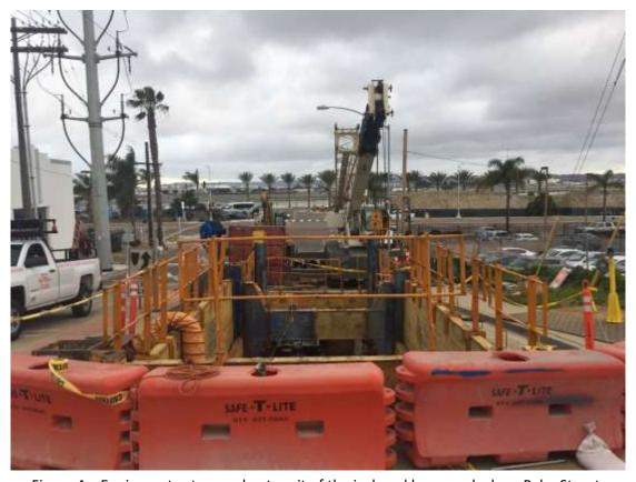
Figure 4 – Equipment set up and entry pit of the jack and bore work along Palm Street.
