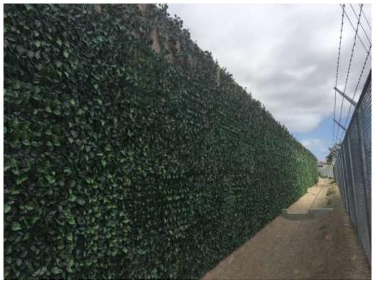
Figure 2 – Artificial ivy installation was installed on the outside western perimeter wall to prevent graffiti.
