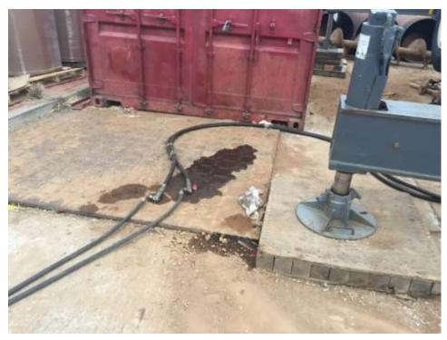
Figure 5 – Leaking hydraulic hoses at the jack and bore site with no spill containment as observed on May 17.
