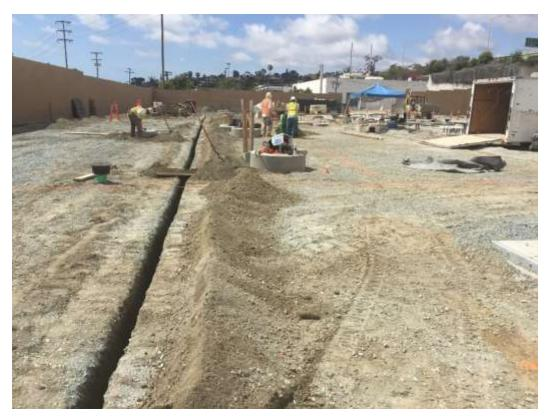
Figure 1 – DCX crews continued with the installation of the substation ground grid.
