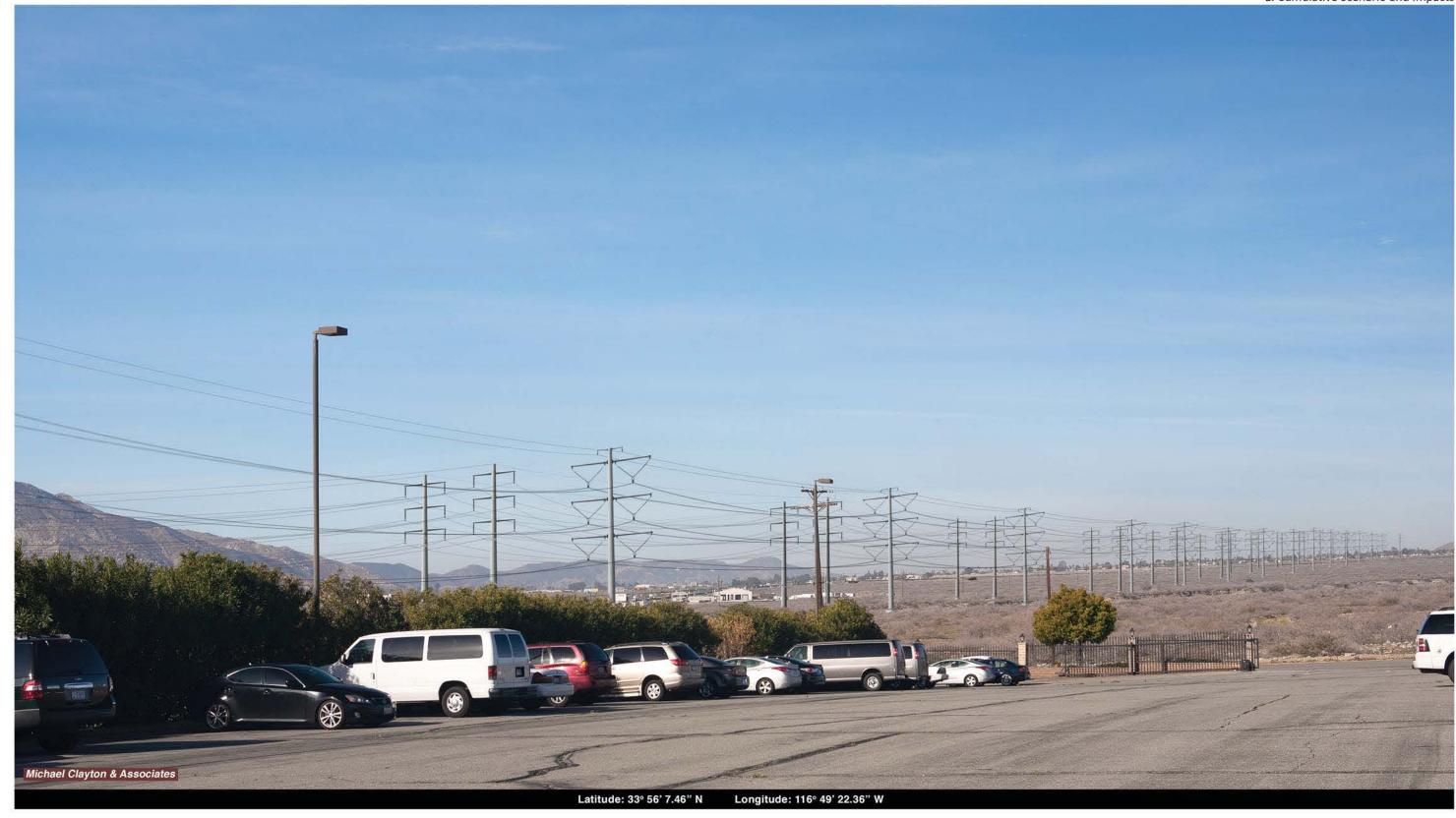
This image presents a **Visual Simulation** of the **Proposed Project plus a Future 500 kV Transmission Line** (cumulative project) from **KOP 12**, at the **Morongo Community Center**. This simulation illustrates the addition of a future 500 kV tubular steel pole transmission line adjacent and to the north of the Proposed Project in the proposed new ROW. The 500 kV structures would be approximately the same height as the 220 kV structures in Segment 5 due to airspace restrictions.
