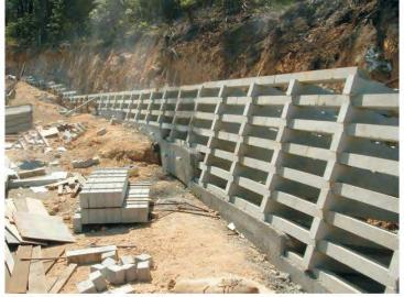
Typical concrete crib wall.
