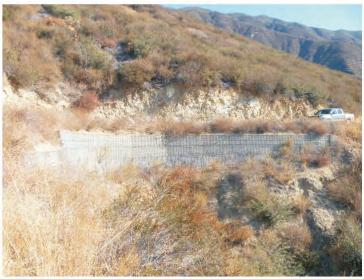
Typical welded wire wall.
