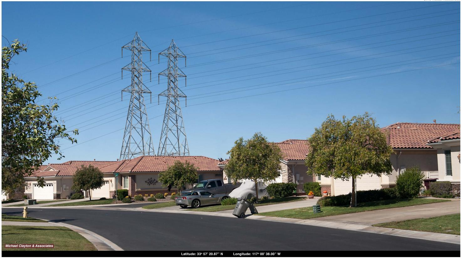
This image presents a **Visual Simulation** of the Proposed Project from **KOP 6A** on Sagura Road, in the Solera residential golf community in the City of Beaumont. This simulation illustrates the replacement of three existing transmission lines with two transmission lines consisting of substantially taller structures. As shown in the simulation, the new structures would appear visually dominant due to their greater heights and close proximity to residences along the south side of the ROW.
