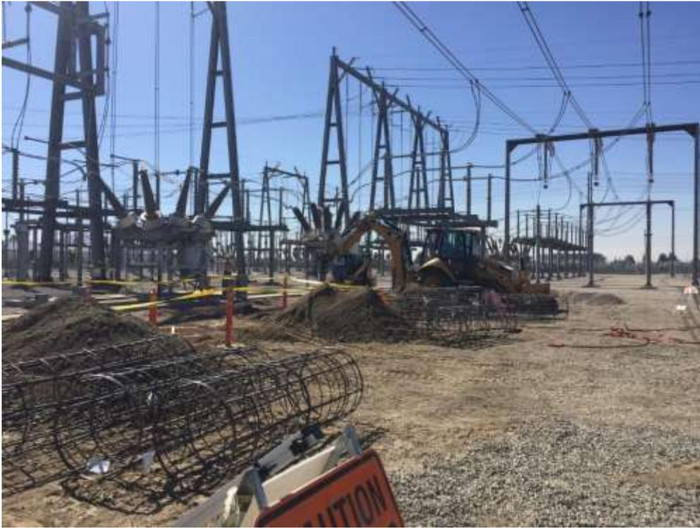
Figure 1 – Construction crews removed existing foundations and drilled holes for new foundations for the replacement switch racks.
