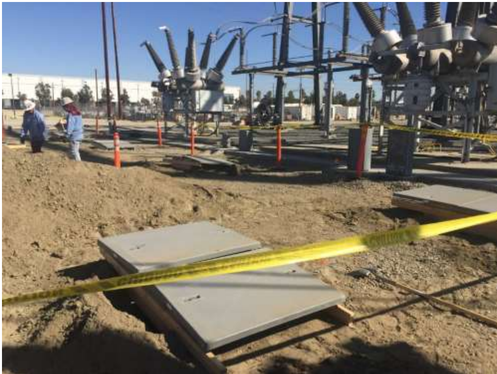
Figure 4 – Foundation holes left overnight are covered to prevent wildlife entrapment.
