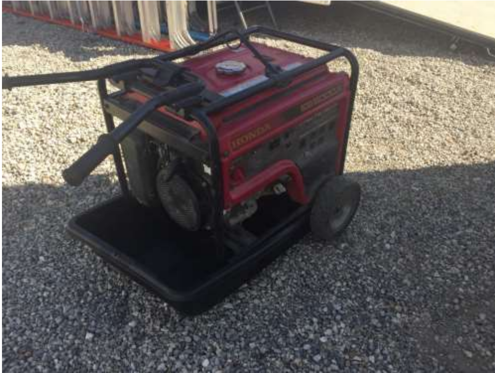
Figure 3 – Drip pans are placed under stationary equipment and under heavy equipment at the end of the day.
