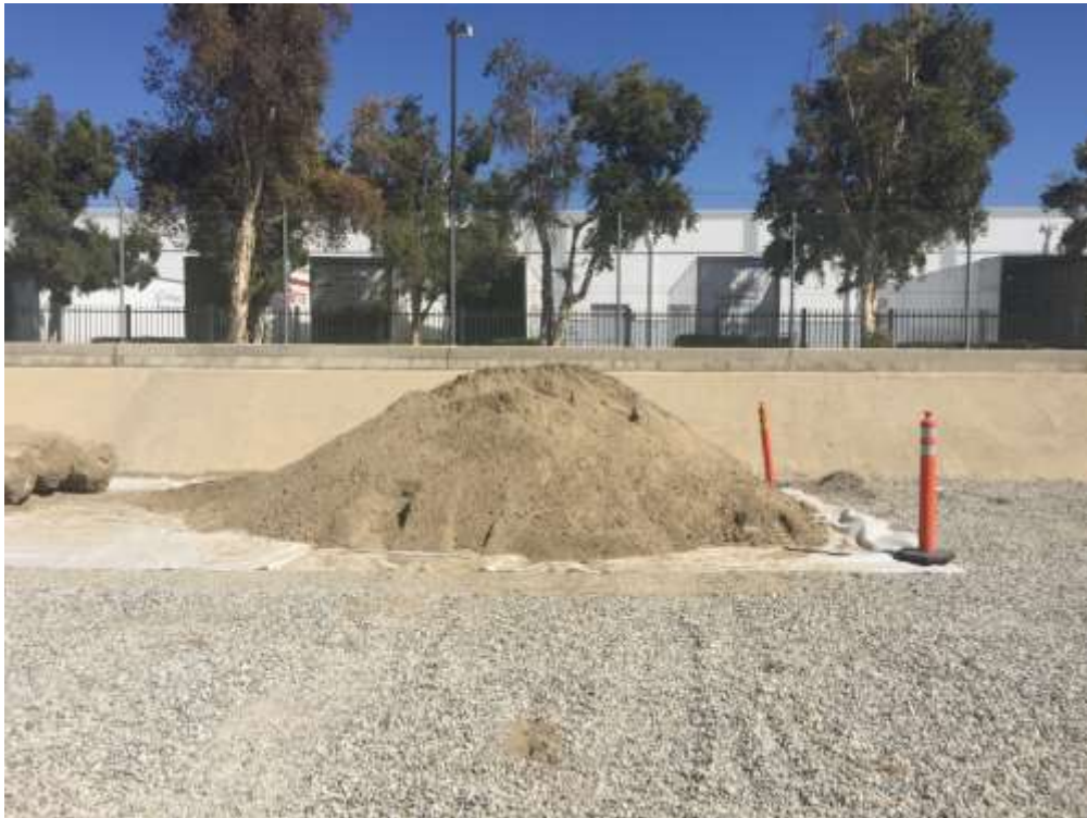
Figure 2 – Soil from foundation excavations is temporarily stored on site until haul
