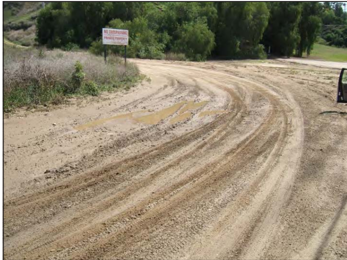
PHOTOGRAPH 1: View looking southeast, showing feature A1. (S. Spencer, 3/26/2012)
