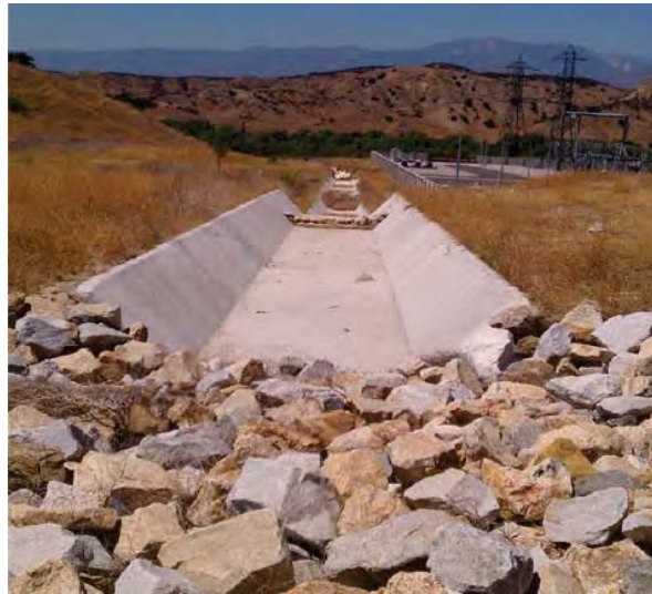
Concrete and rip rap channel. These areas may have Corps jurisdiction if they replace an historical drainage and if they connect to a drainage with a connection to a traditional navigable water.
