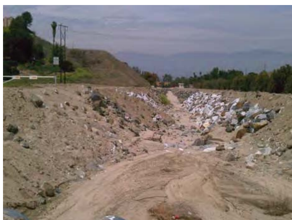
Reche Canyon, a trapezoidal earthen and rip rap channel east of the City of Grand Terrace that is potentially jurisdictional for CDFG and Corps.
