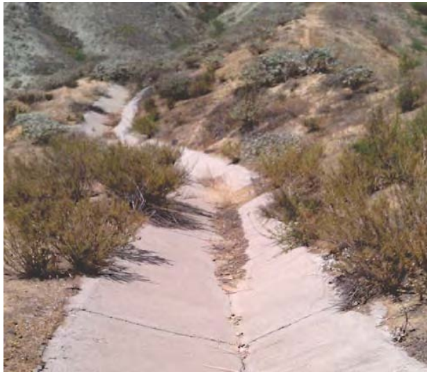
Concrete v-ditch. These areas are often erosion control features excavated on dry land, with no value for fish and wildlife resources. As such they are usually not Corps or CDFG jurisdictional. If they replace a natural drainage or convey flow from one natural drainage to another they are likely CDFG jurisdictional and, Corps jurisdictional, if they connect to a drainage with a connection to a traditional navigable water.
