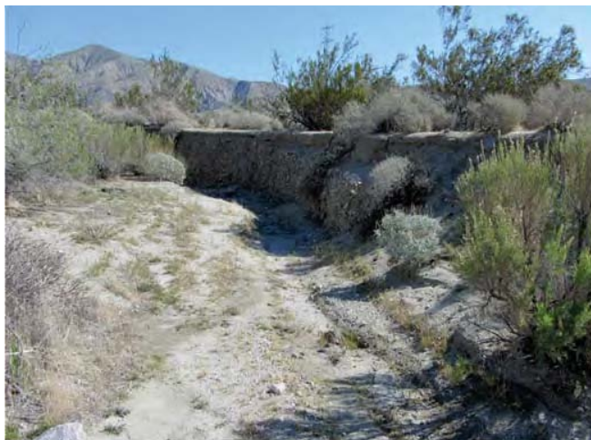
Ephemeral channel with clear evidence of change in particle size distribution, benches, and exposed roots. This drainage is both potentially CDFG and Corps jurisdictional.
