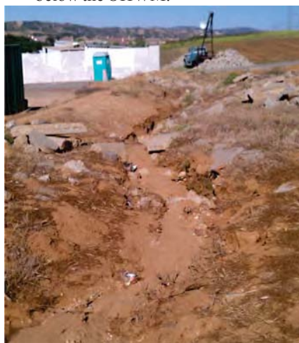
Ephemeral channel showing change in particle size and lack of vegetation at/below the OHWM.
