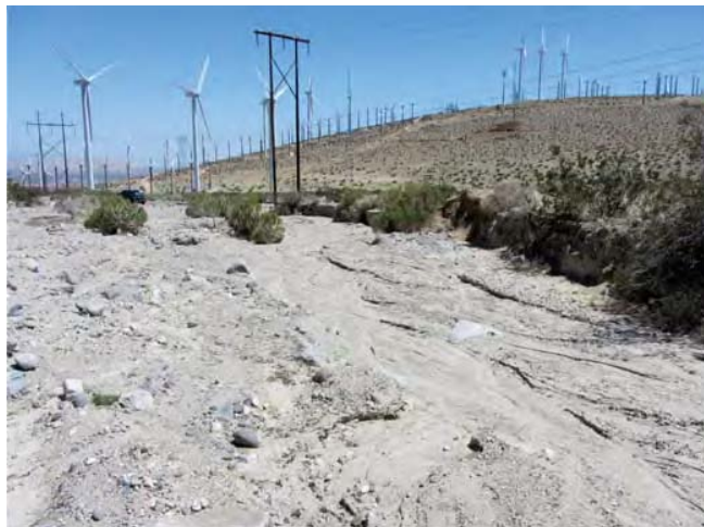
Super Creek shows evidence of change in particle size distribution, benches, and exposed roots. This drainage is both potentially CDFG and Corps jurisdictional.
