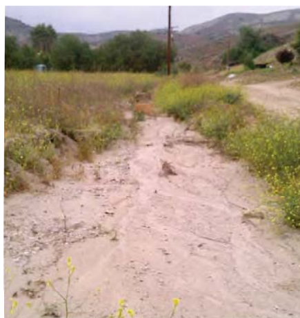
Roadside wash that conveys flows with evidence of gravel sheets (sand ridges) below the OHWM.
