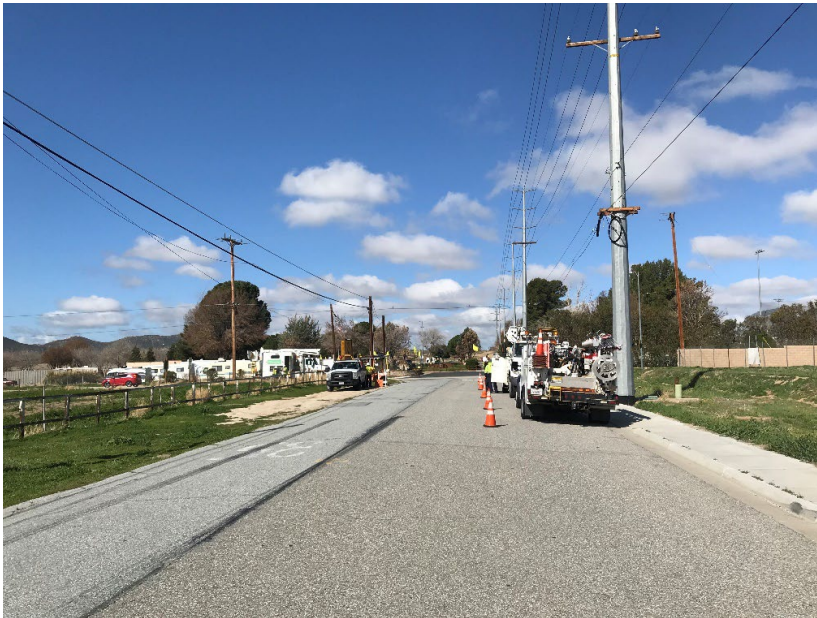
Photo 3. SCE crew splicing fiber along Wesley Avenue (March 26, 2018)
