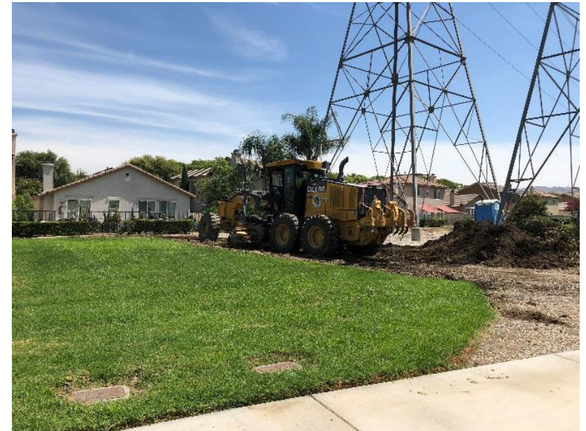
Photo 4. Vegetation removal occurring at Site 1X12-1X13 along Segment 1 (August 28, 2018)
