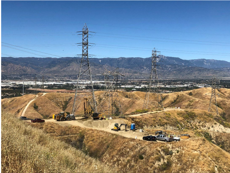
Photo 5. Grading and drilling occurred in Segment 2 (April 24, 2019)
