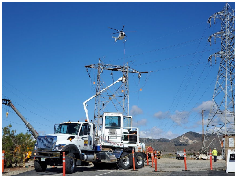
Photo 9. Wire wreck-out activities at Construction Area 5X29, Segment 5 (March 11, 2020)
