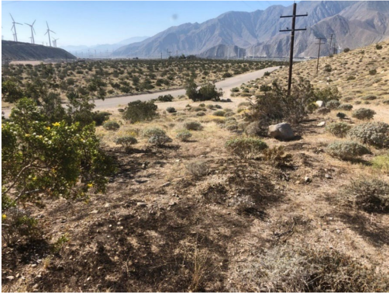
Photo 13. Fire damage caused by dropped wire striking a distribution line between Construction Areas 6N27 and 6N28, Segment 6 (May 1, 2020)
