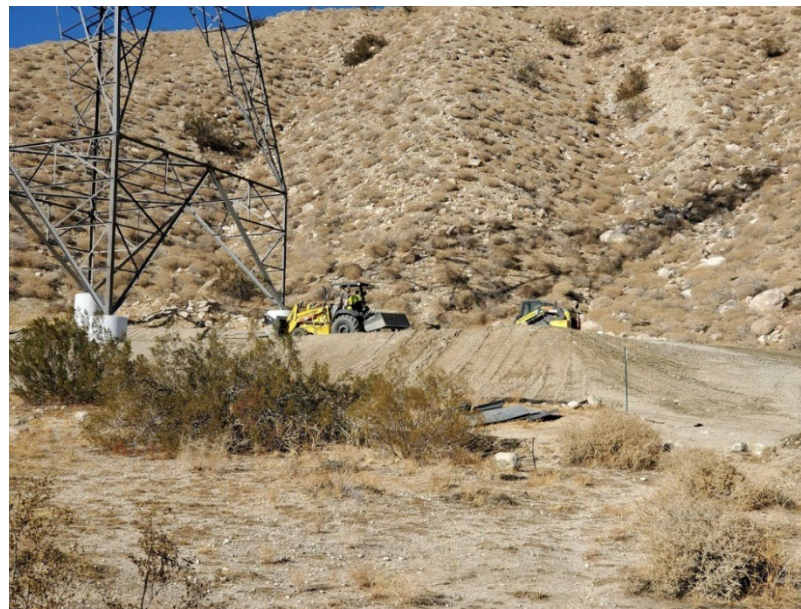
Photo 10. Site restoration activities at Construction Area 6531A, Segment 6 (December 21, 2020)
