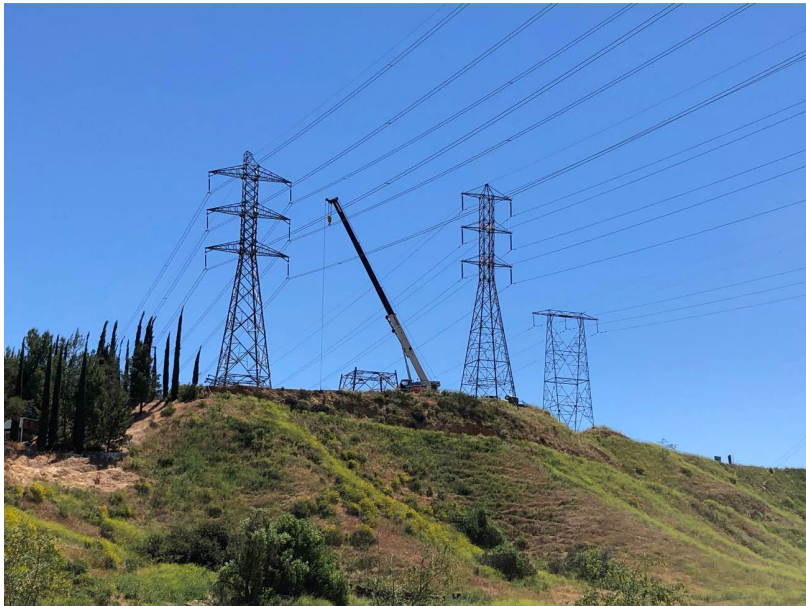
Photo 7. Tower assembly activities occurred in Segment 3 (April 23, 2019)
