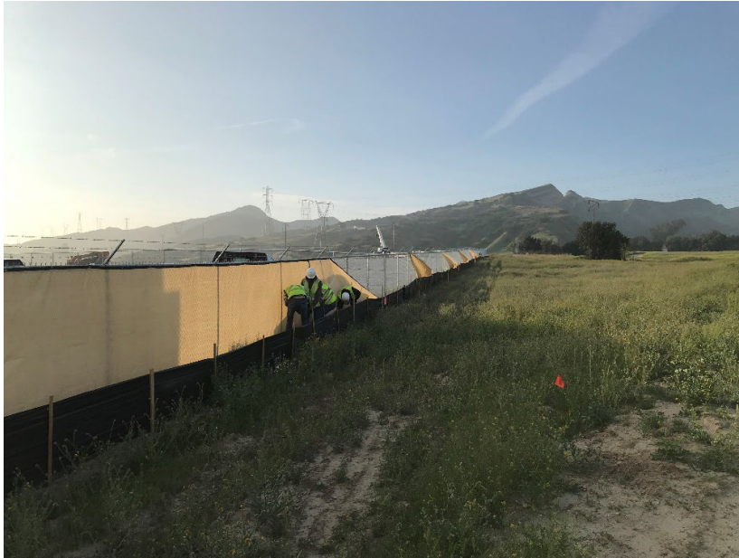
Photo 1. Installing privacy screening around perimeter of Poultry MY (April 4, 2018)
