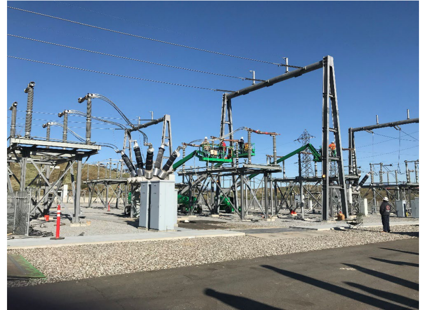
Photo 2. Crews working at bus position #7 at El Casco Substation (March 27, 2018)
