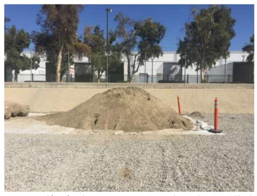
Figure 2 – Soil from foundation excavations is temporarily stored on site until haul
