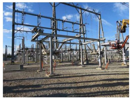
Figure 1 – Construction crews installed the new switchracks on the northern portion of the work area, October 11, 2017.
