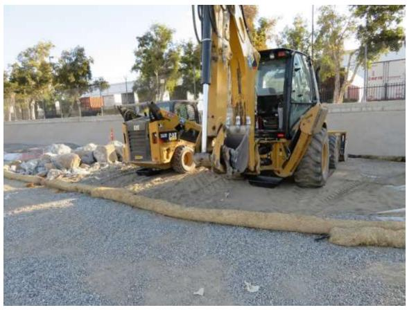
Figure 3 – Straw wattles were installed around the remaining soil stockpile in the material storage area, October 11, 2017.
