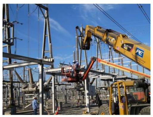
Figure 2 – New insulators were installed on the new switchracks, October 11, 2017.
