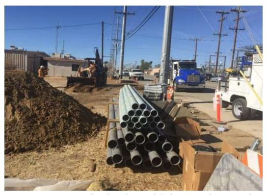
Figure 2 – W.A. Rasic crew conducted trenching, manhole placement, and saw-cutting along Lincoln Street on December 7, 2017, Banning Substation Telecommunications alignment.
