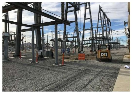
Figure 1 – Pouring foundations for disconnect replacement of the Mountain View #3 Line at San Bernardino Substation on November 30, 2017.
