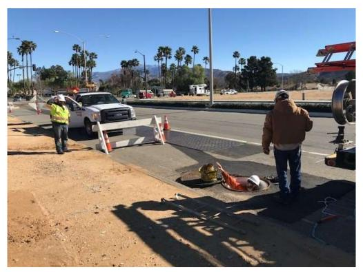
Figure 1 – SCE crew installing innerduct at intersection of East First Street and Highland Springs Avenue (January 22, 2018).
