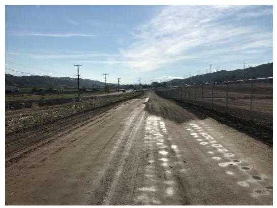
Figure 3 – Installation of rock base along main access road to Poultry MY (March 9, 2018).
