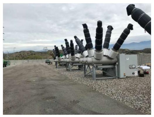
Photo 5 – New bus positions onsite and ready for installation at the El Casco Substation (March 21, 2018).
