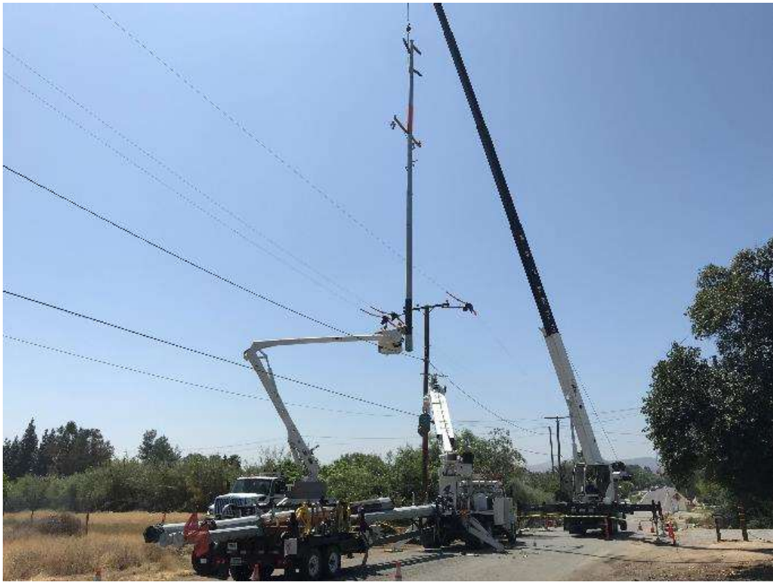
Photo 5 – Installation of TSP along Nevada Street for Tennessee Relocation (May 9, 2018).
