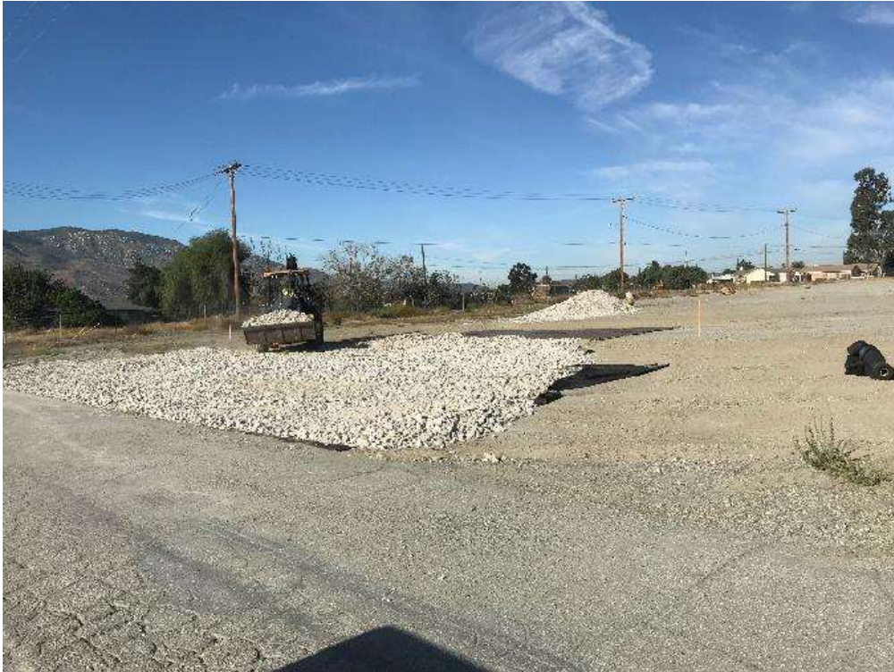
Photo 1 – Installing rock base BMP to stabilize entrance at Match MY (May 9, 2018).
