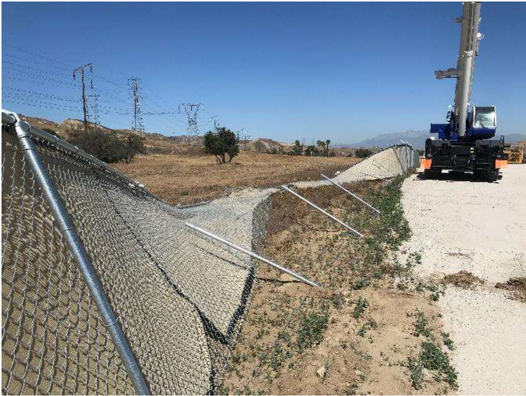
Photo 3 – Damaged chain link fencing and privacy screening due to theft at Poultry MY (May 7, 2018).
