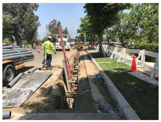
Photo 4 – Trenching for underground conduit at Barton Road and Iowa Street for Tennessee Relocation (May 14, 2018).
