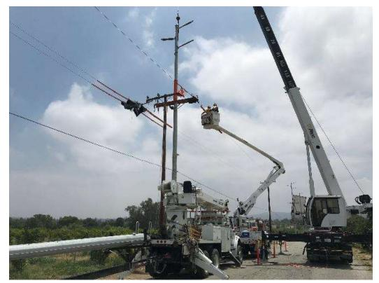
Photo 4 – Installing LWTSP at Iowa Street and Citrus Street for Tennessee Relocation (May 24, 2018).
