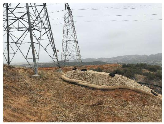
Photo 8 – Topsoil properly covered and maintained for salvage at Tower Site 4X55 (May 24, 2018).
