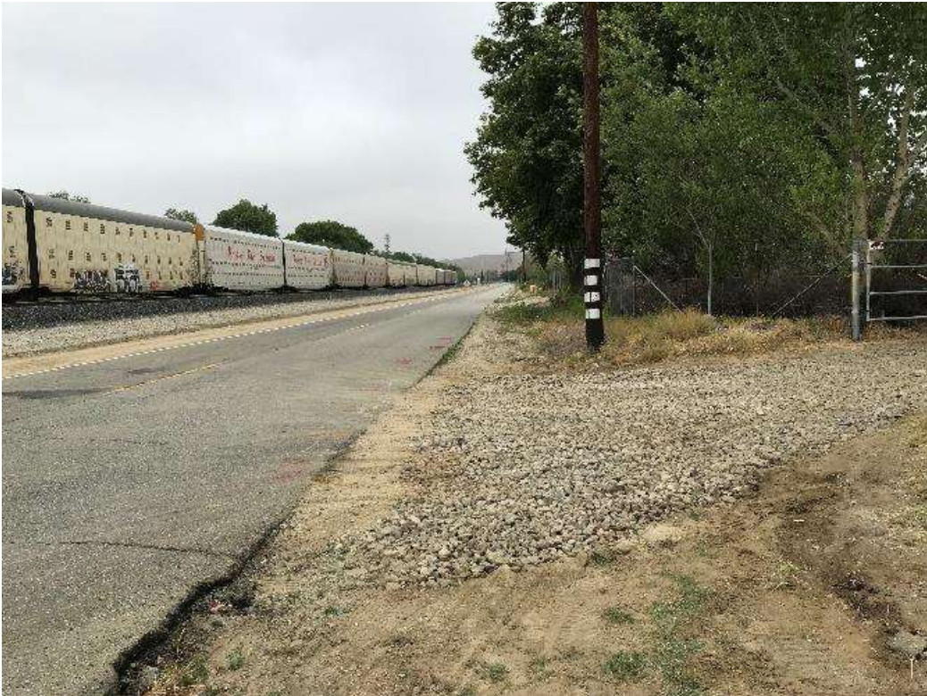
Photo 6 – Adequate entrance stabilization and trackout control along San Timoteo Canyon Road (May 30, 2018).
