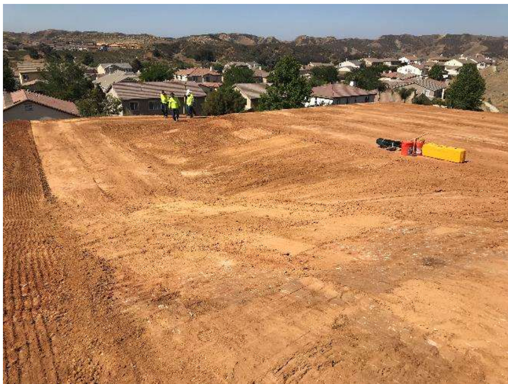
Photo 4 – Grading activities completed at Tower Site 4X53 (June 8, 2018).
