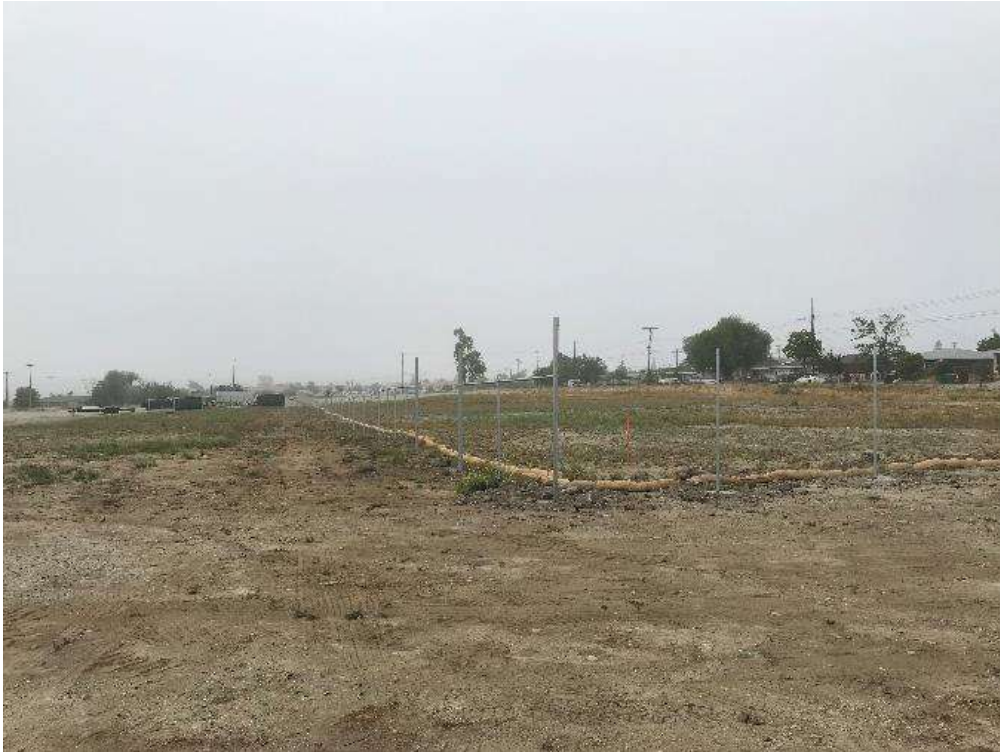
Photo 1 – Installing poles for perimeter chain link fencing at Match MY (May 30, 2018).
