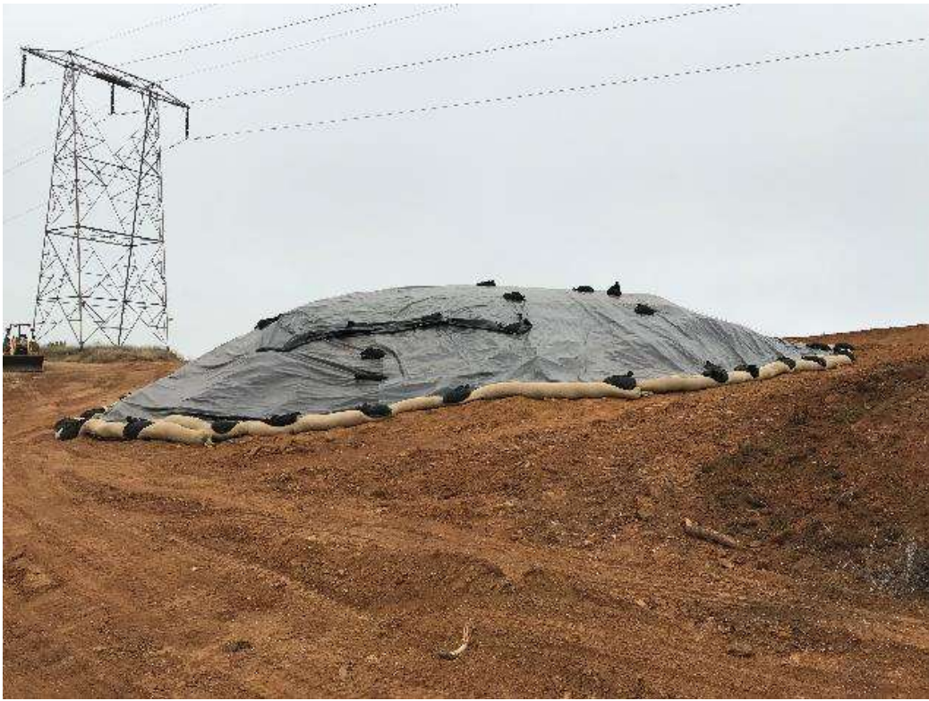
Photo 5 – Soil stockpile properly contained at Tower Site 4X51 (May 30, 2018).
