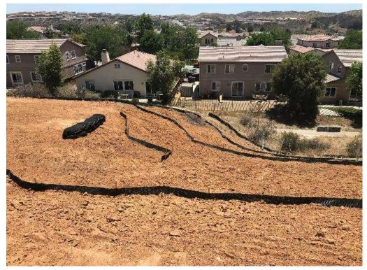
Photo 5 – BMPs installed to contour at Tower Site 4X53 (June 12, 2018).
