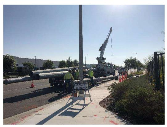
Photo 3 – Installing LWTSP at intersection of Lugonia Avenue and Bryn Mawr Avenue for the Timoteo Relocation (June 26, 2018).
