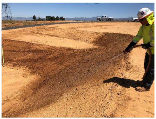
Photo 5 – Applying BMP (soil stabilizer) to slopes at Tower Site 4X47 (June 25, 2018).
