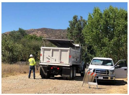
Photo 8 – Haul truck properly covering load and construction crew sweeping outside bed of truck to minimize trackout along San Timoteo Canyon Road (June 26, 2018).
