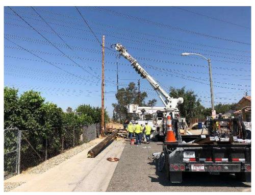
Photo 2 – Installing a new wooden pole along Juanita Street for Juanita Reconductor (June 29, 2018).
