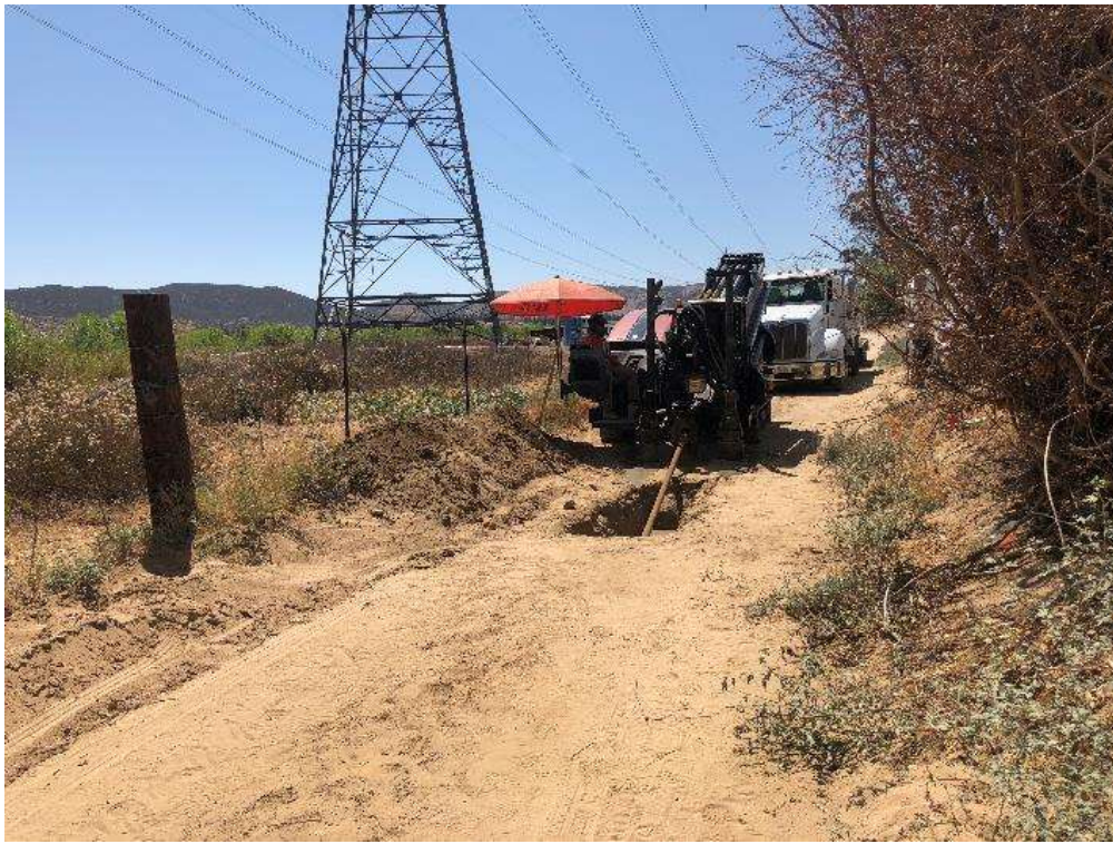
Photo 3 – HDD operations occurring along Smith Creek for the Banning Connection (August 14, 2018).
