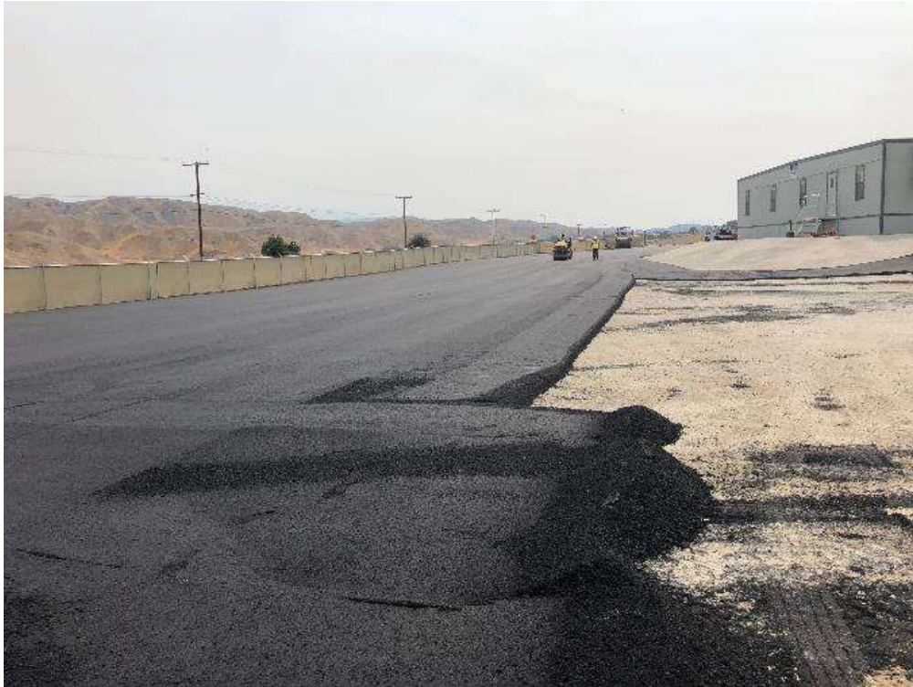
Photo 1 – New pavement being applied at Poultry MY (August 10, 2018).
