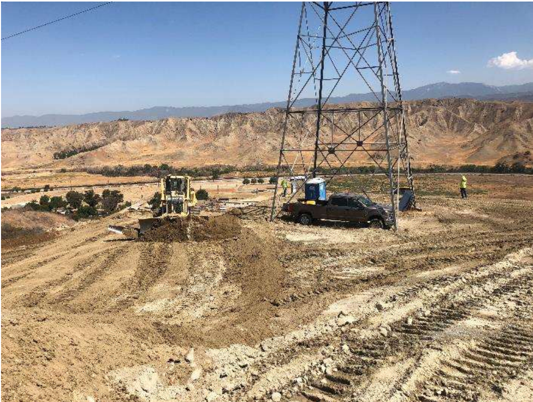
Photo 8 – Grading activities occurring at Site 3X19 (August 14, 2018).
