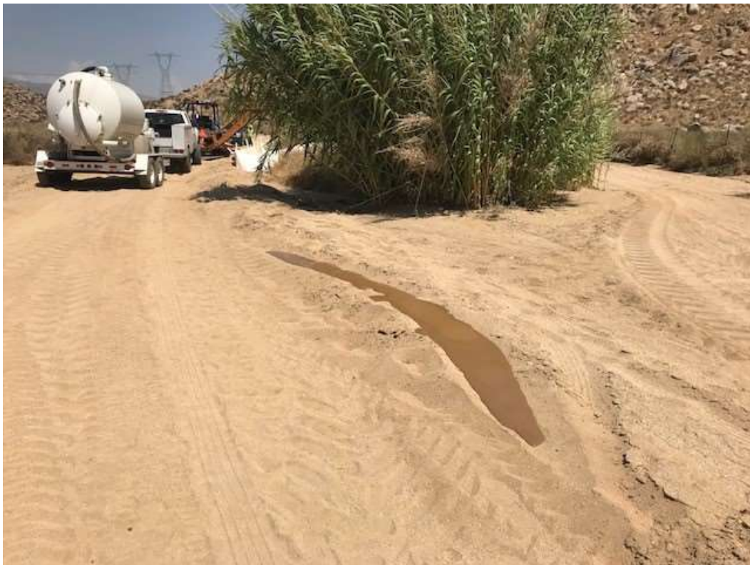
Photo 6 – Initial frac-out identified by CPUC EMs along Smith Creek during HDD operations (August 14, 2018).
