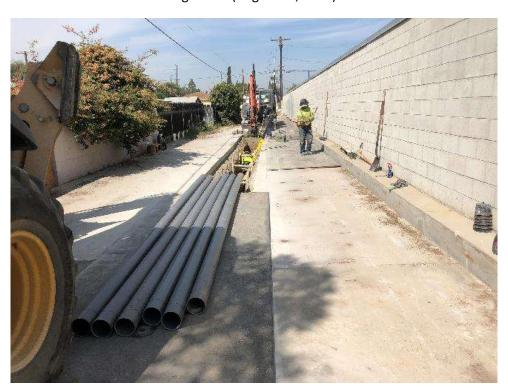
Photo 2 – Trenching and installing underground conduit along the Timoteo Relocation (August 28, 2018).
