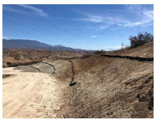
Photo 6 – Mid-slope BMPs properly installed at Site 3X19 along Segment 3 (August 30, 2018).
