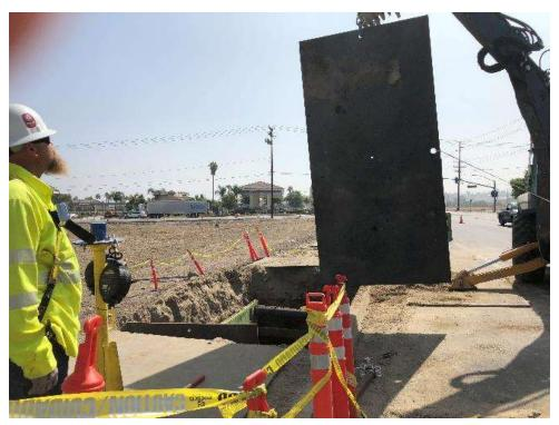
Photo 1 – Excavating underground vault along the Dental/Intern Circuit alignment (August 27, 2018).
