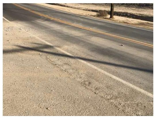
Photo 7 – 4-inch rock tracked onto San Timoteo Canyon Road from a stabilized entrance to Site 3X33 (September 20, 2018). The track out was attributed to another utility working on an unrelated project, but the BMP was installed by the West of Devers Project and will be maintained or removed.
