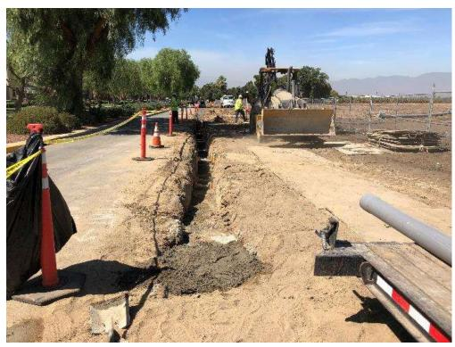
Photo 1 – Trenching and conduit installation along Mission Avenue for the Dental/Intern Circuits (September 26, 2018).
