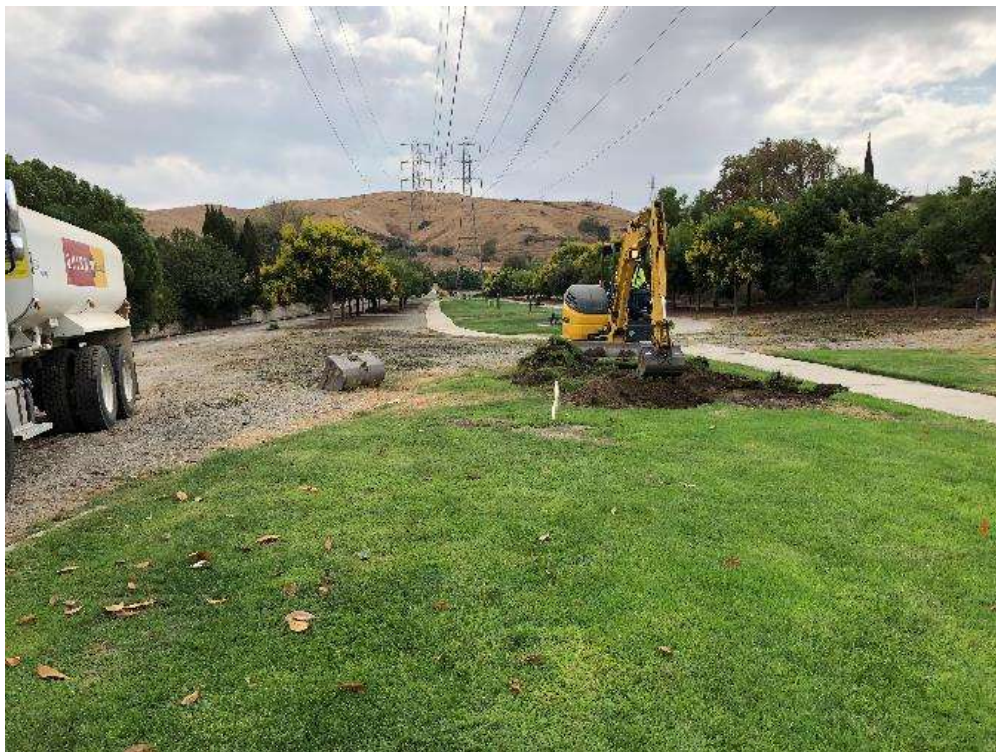
Photo 2 – Power Grade crew removing vegetation at Site 1X04-1X05, Segment 1 (October 2, 2018).
