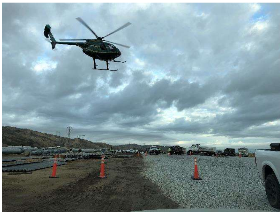
Photo 4 – Summit Helicopter vessel landing at Poultry MY in preparation of wire stringing activities along Segment 4 (October 3, 2018).
