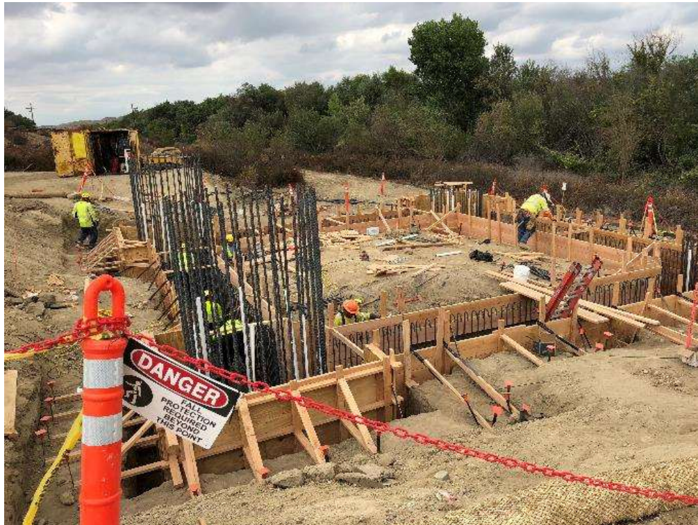
Photo 3 – Installing forms for grade beam at Site 4N64, Segment 4 (October 2, 2018).
