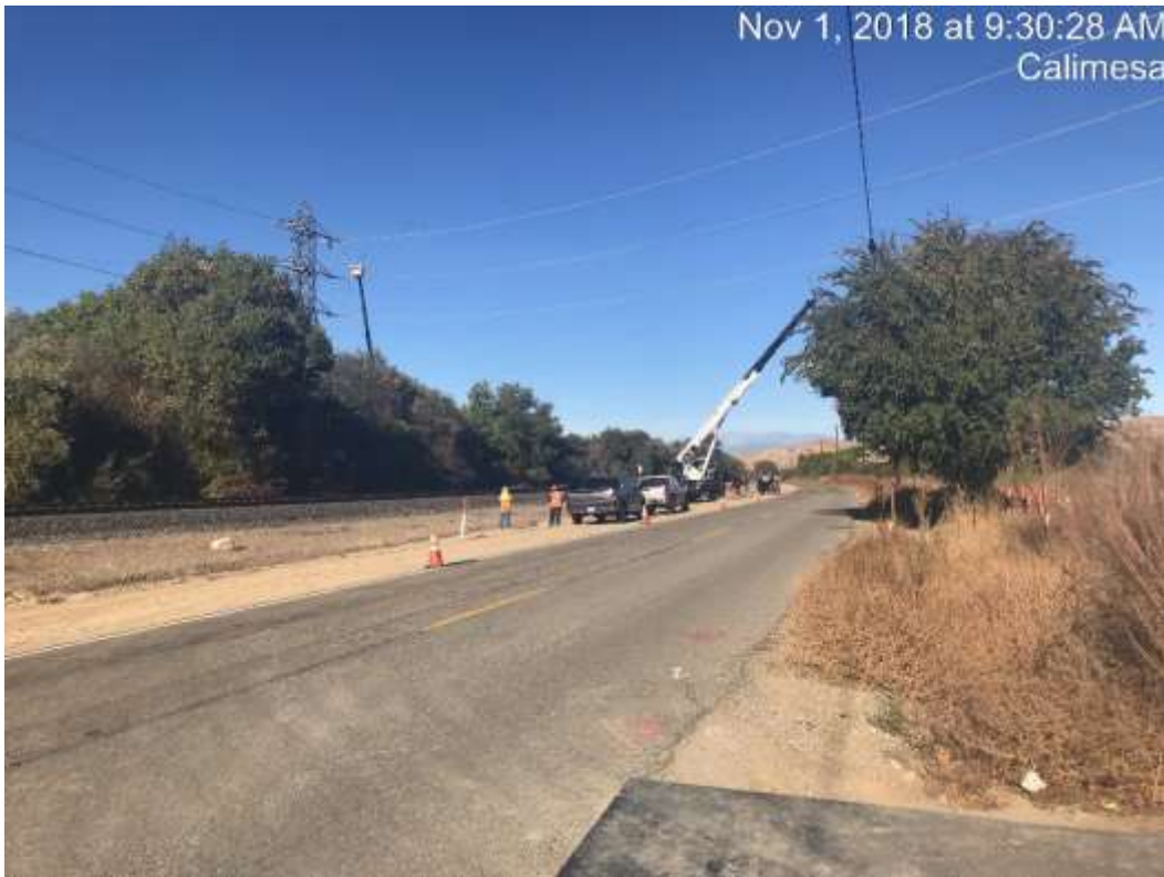
Photo 4 – Wire stringing across San Timoteo Road, Segment 4 (November 1, 2018).
