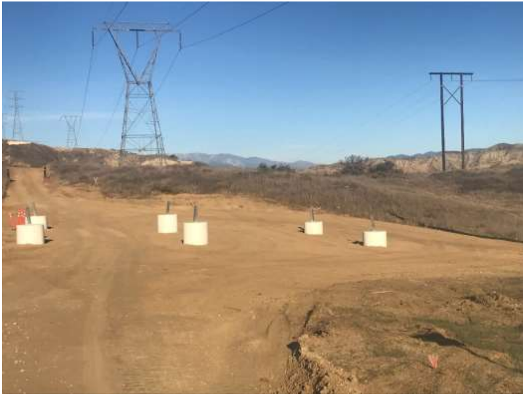
Photo 3 – Completed foundations at Segment 3 Tower 3X14 (October 31, 2018).
