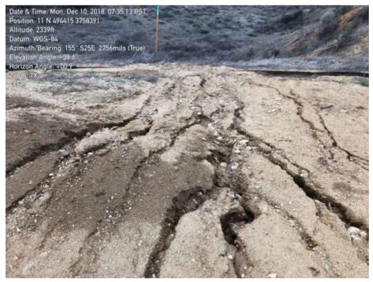
Photo 3 – Erosion observed at Tower 57, Segment 4 after the prior week's storm. Photo courtesy of SCE.
