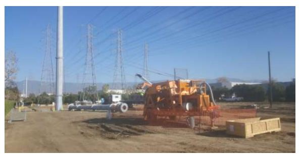
Photo 1 – Wire stringing in Segment 1; part of the current outage work (Move 1).
