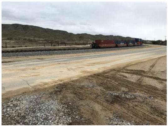
Photo 5 – Track out onto San Timoteo Canyon Road and the stabilized construction entrance to Site3X22, Segment 3. A sweeper was dispatched to clean up the street and maintenance of the stabilized entrance included addition of more rock.
