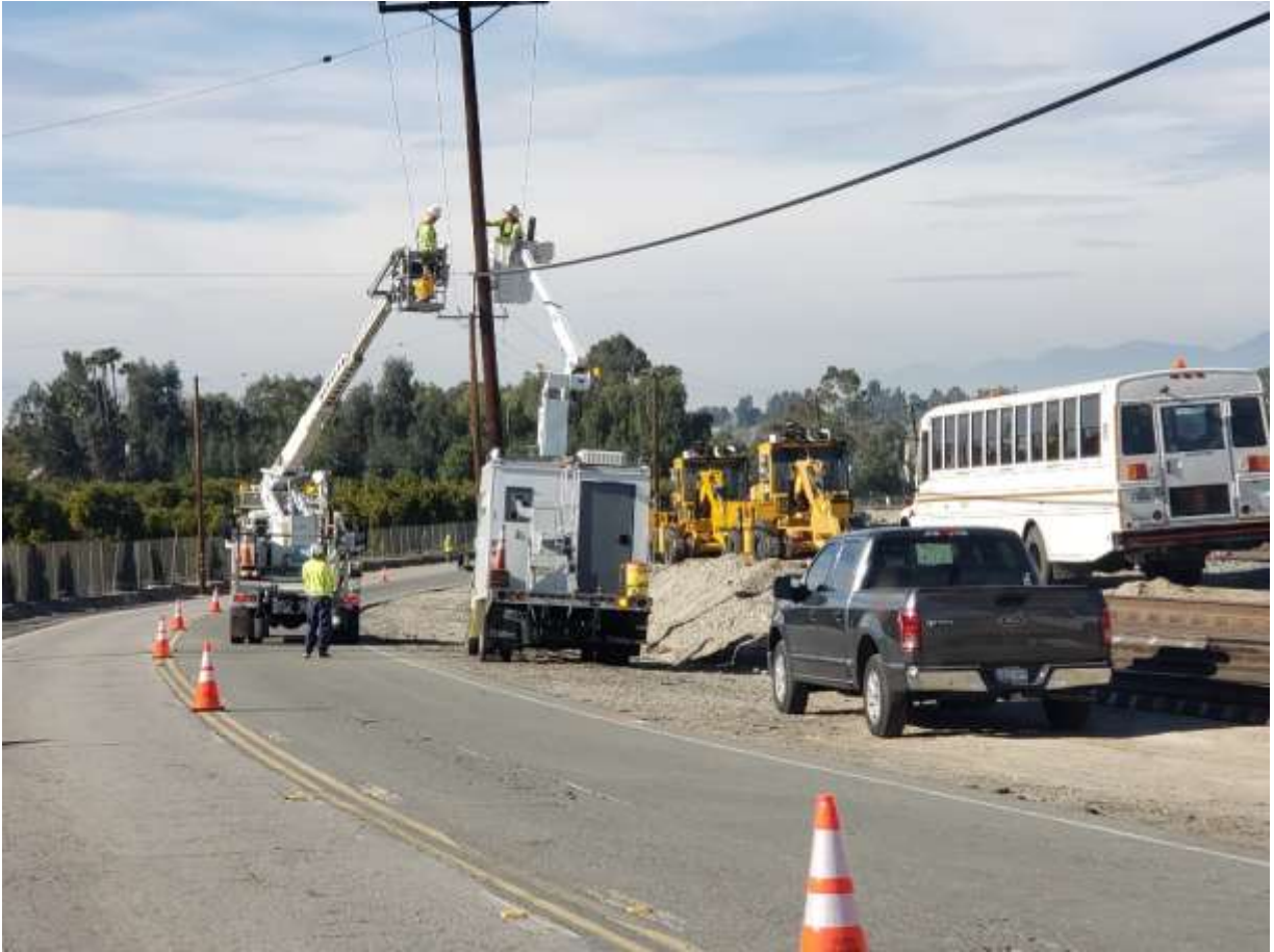
Photo 1 – SCE Telecom work along San Timoteo Canyon Road.
