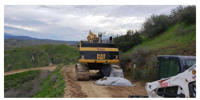
Photo 6 – Tracks of excavator covered to contain hydraulic fluid as a result of a reportable spill along the access road between Sites 3X37 and 3X38 (Segment 3; February 13, 2019).
