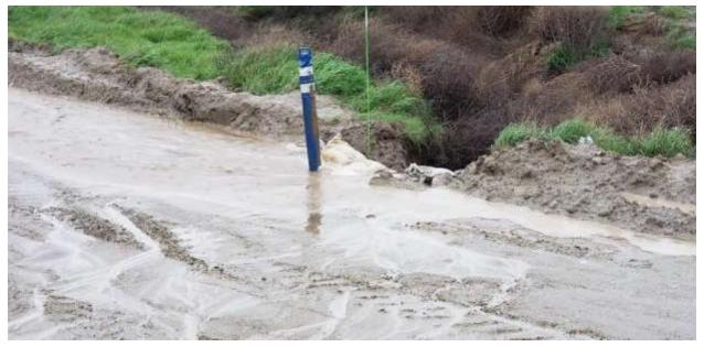
Photo 4 – Offsite sedimentation into jurisdictional feature along the access road to Site 3X06-07 (Segment 3; February 14, 2019).
