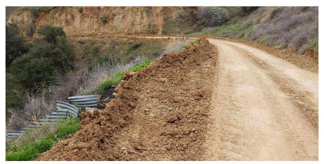
Photo 5 – MacCarthy drain blocked as a result of grading along Segment 3 access road (Segment 3; February 13, 2019).
