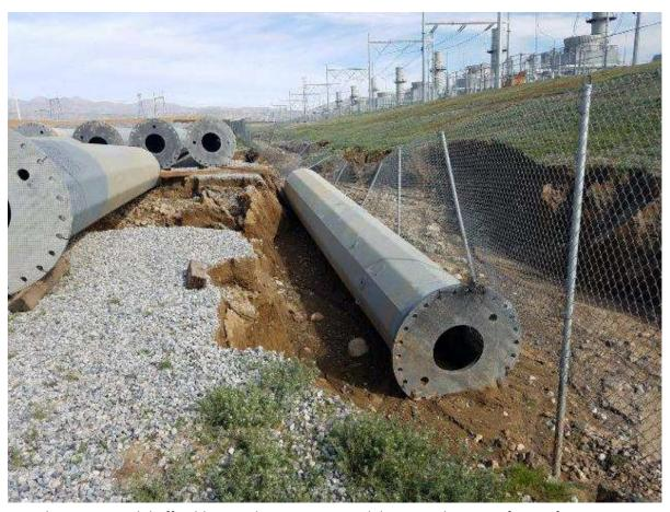
Photo 1 – TSP slid off cribbing and into unapproved drainage along east fence of Devers MY (February 15, 2019) (photo courtesy of SCE).
