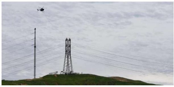
Photo 2 – Wire stringing activities between Site 3N02 and El Casco Substation (Segment 3; February 12, 2019).
